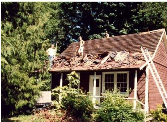
Removing old shingles in 1989 re-roofing project
