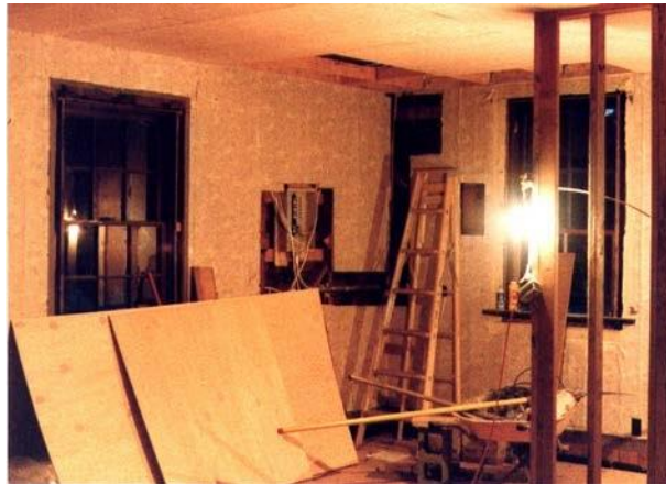
Interior repairs in 1982 after School House moved to the heritage site
