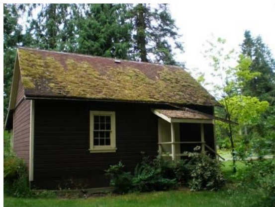
Rear of School House prior to second shingling in 2007
