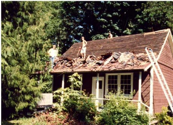
Removing old shingles in 1989 re-roofing project
